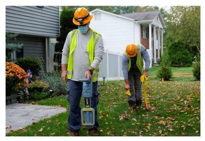
PHOTO CAPTION: Two O&R damage prevention technicians team up to locate and mark out underground O&R gas and electric facilities at a home in Nanuet. In the foreground James Misczuk uses a radio detection receiver to locate O&R underground gas facilities while J.D. Gallo follows to mark the locations with paint and flags. This procedure warns excavators to avoid digging near the facilities.
